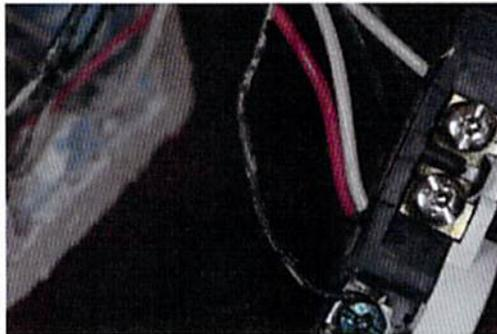
Black corrosion on wiring
