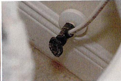
Corroded shut off valve
